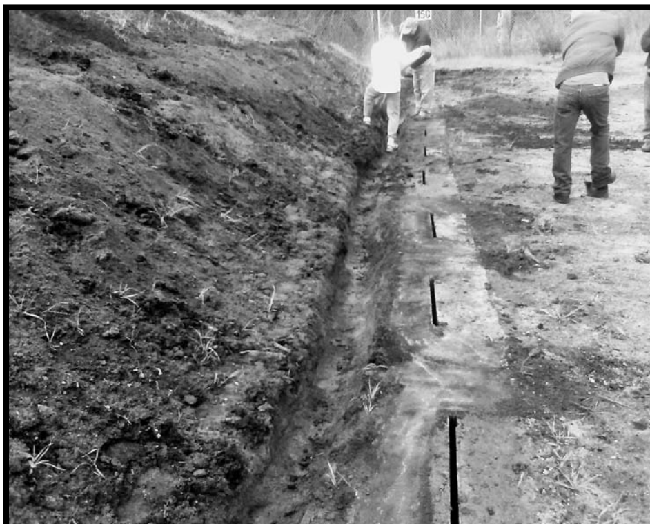
Work party, does repairs on the 150 yrd range, February 15, 2009
