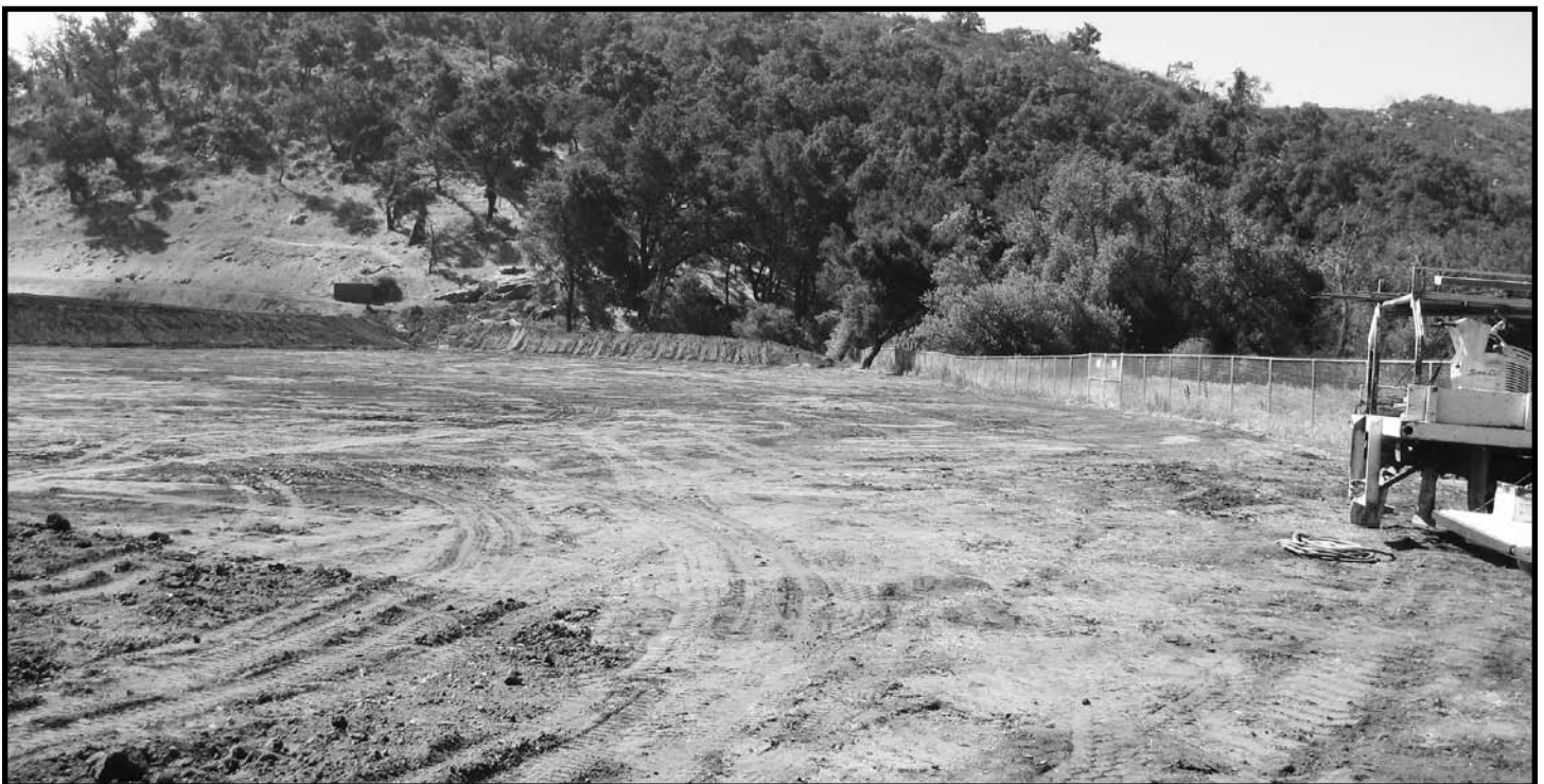
New Rifle Range Under Construction.
